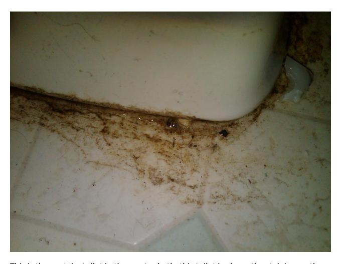
This is the upstairs toilet in the master bath, this toilet is above the staining on the ceiling in the room just below it. I flushed this toilet and water poured out from under it with just one flush. The ceiling just below this has a couple of areas that are close to the toilet and the shower in this room and both have issues with water coming out from under as in this picture.
