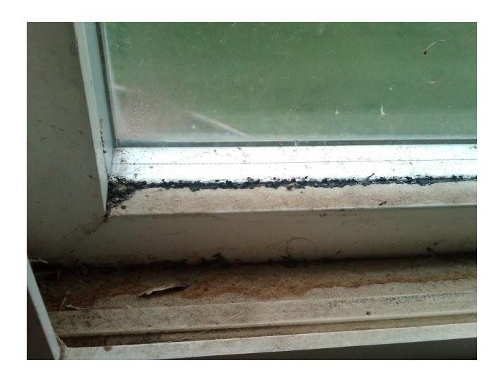
The black where the window meets the plastic is full of water. And you can see where water had run down and onto the inside of the window trim.
