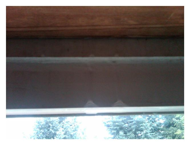
This picture is from the inside of the slider, looking out to the back yard. You can see at the top water running down the plastic trim from up above the wood area.
