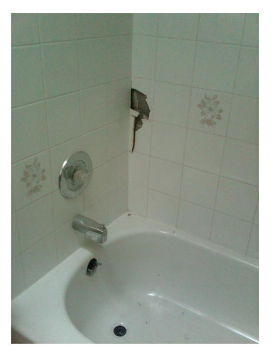
This is the same bathtub on the hallway side. You can see the tub drain cover missing and also the overflow cover. There is also a large hole in the wall. The tile is missing. If anyone took a shower in this tub it would get the ceiling wet in the room just below it. I checked the ceiling below this and the master bath and I did not get any moisture readings. The staining was from a while ago.
