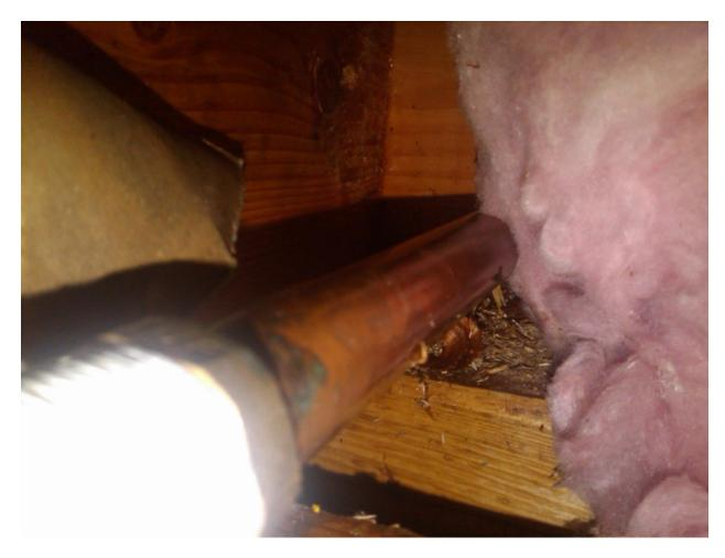
This picture is of the frost free hose bib to the front yard. It has a crack in it from being frozen. You can see a small amount of water running down it in this picture. If the homeowner turns this faucet on, it will run at full strength and most of it will run inside of the house and down onto the floor and all over the ceiling.
