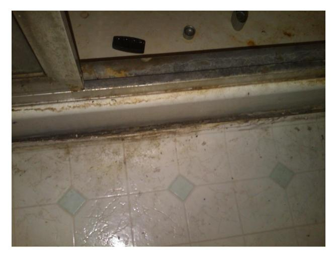
This is still the master bath. The linoleum has separated from the pan by about ½ of an inch. The separation runs almost the whole length of the shower stall. If water were to get between the separations it would go down onto the ceiling in the next room. The area in this picture is close to the marks on the ceiling.
