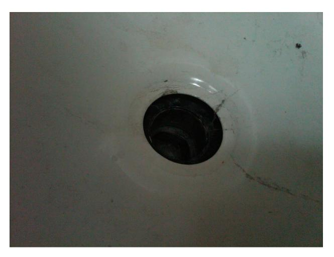
This is the bathtub in the hallway bathroom. The drain is missing the entire cover. If water where to be run down this tub it would flow all over the sub floor and also down onto the ceiling in the same room below the master bath. These bathrooms are back to back.
