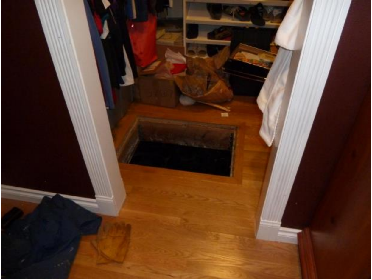
Crawl space opening .
